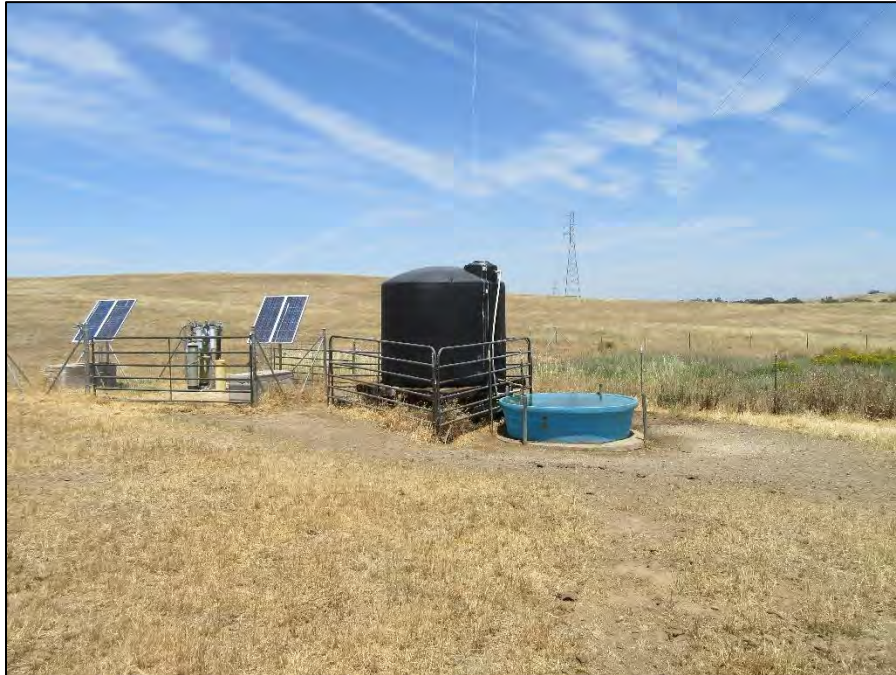
CC-02; well house and modern additions overview (view north; May 27, 2022).
