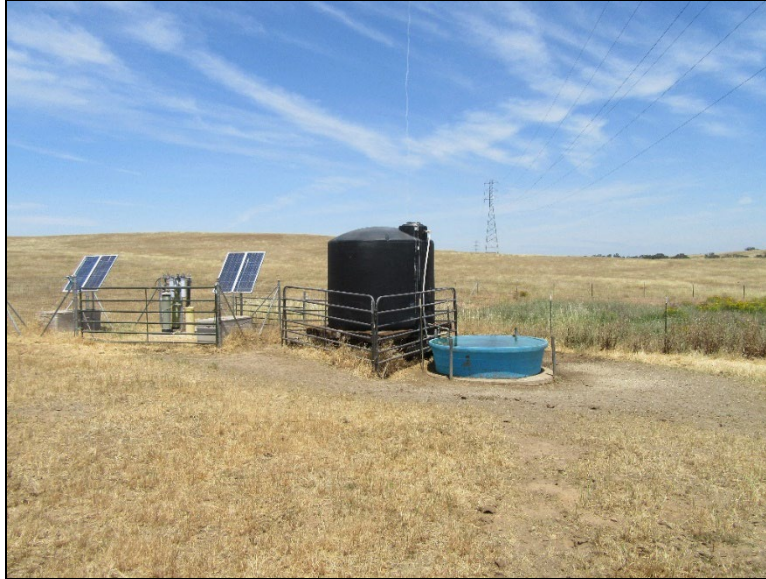
Figure 40. CC-02; Well and Modern Additions Overview (view north; May 27, 2022).
