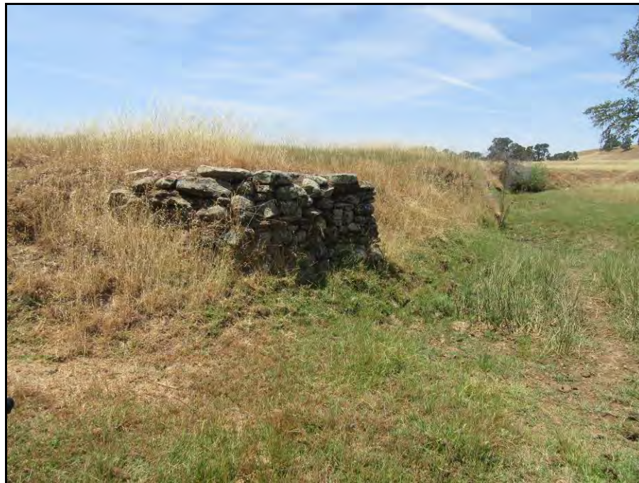
P-34-1575; bridge abutment overview (view northwest; May 27, 2022).
