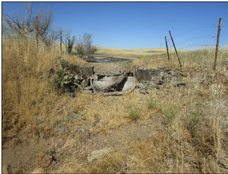
Figure 47. CC-08; Reservoir Overview (view west; June 16, 2022).
