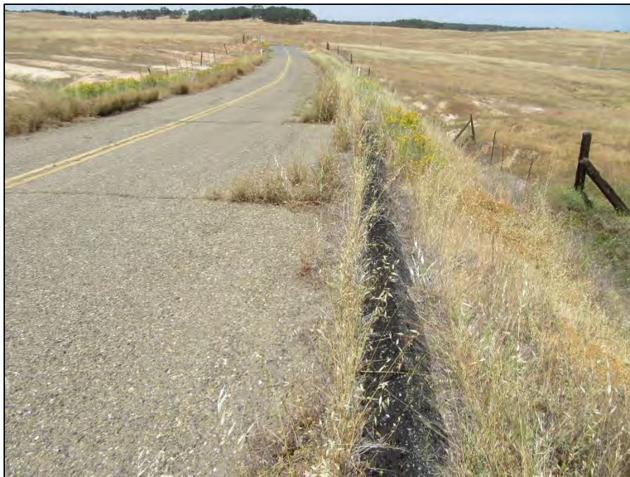
Boys Ranch Road overview (view east; May 27, 2022).
