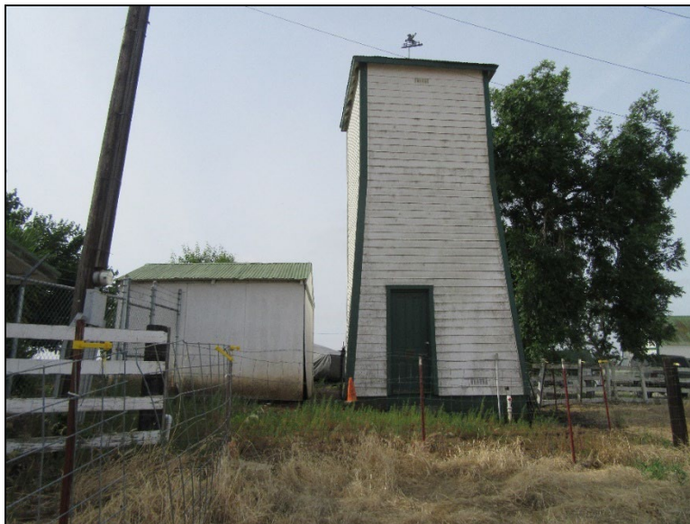
Figure 21. CC-01; Tankhouse (view south; May 27, 2022).
