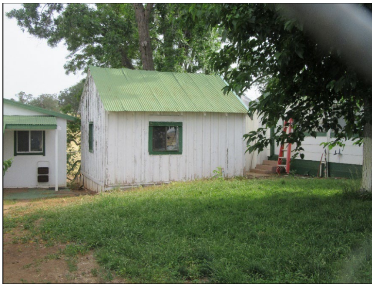
Figure 18. CC-01; Worker's Quarters/Shed (view north; May 27, 2022).
