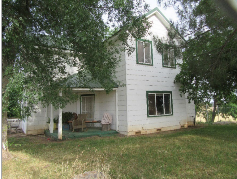
Figure 17. CC-01; Main House (view west; May 27, 2022).
