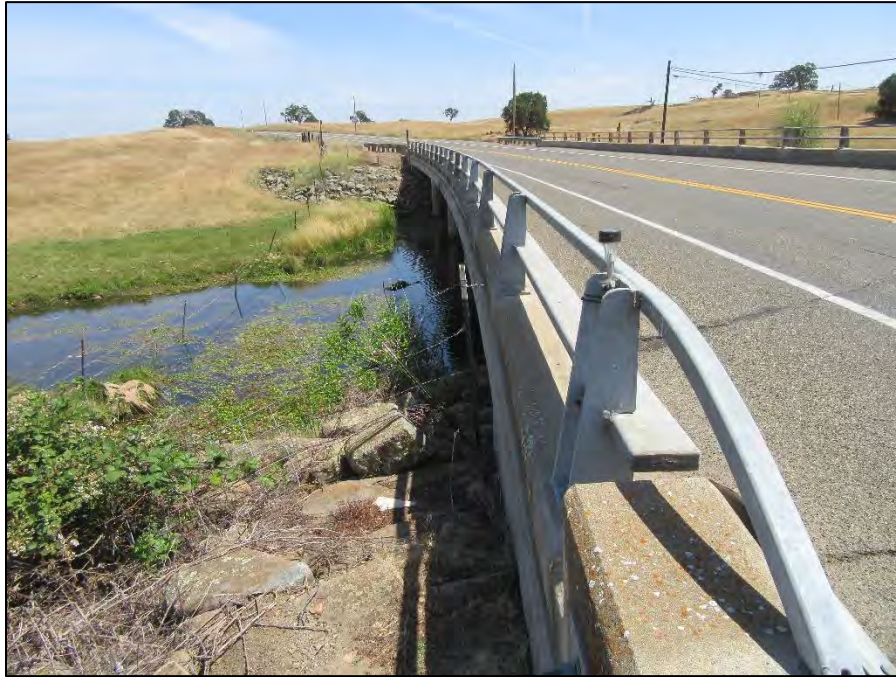
Bridge No. 24C0238 overview (view south; May 27, 2022).
