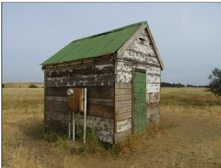
Figure 28. CC-01; Well House (view northwest; May 27, 2022).
