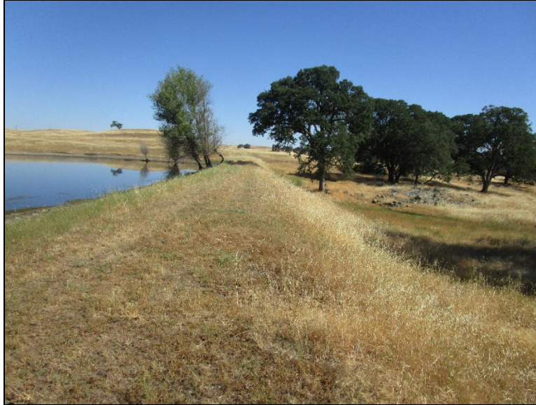
Figure 46. CC-08; Earthen Dam Overview (view north; June 16, 2022).
