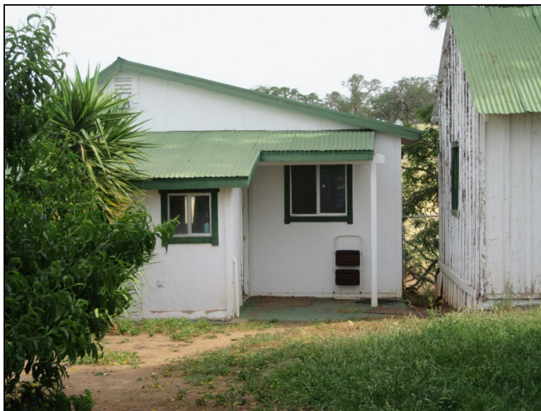
Figure 19. CC-01; Foreman's Residence (view north; May 27, 2022).
