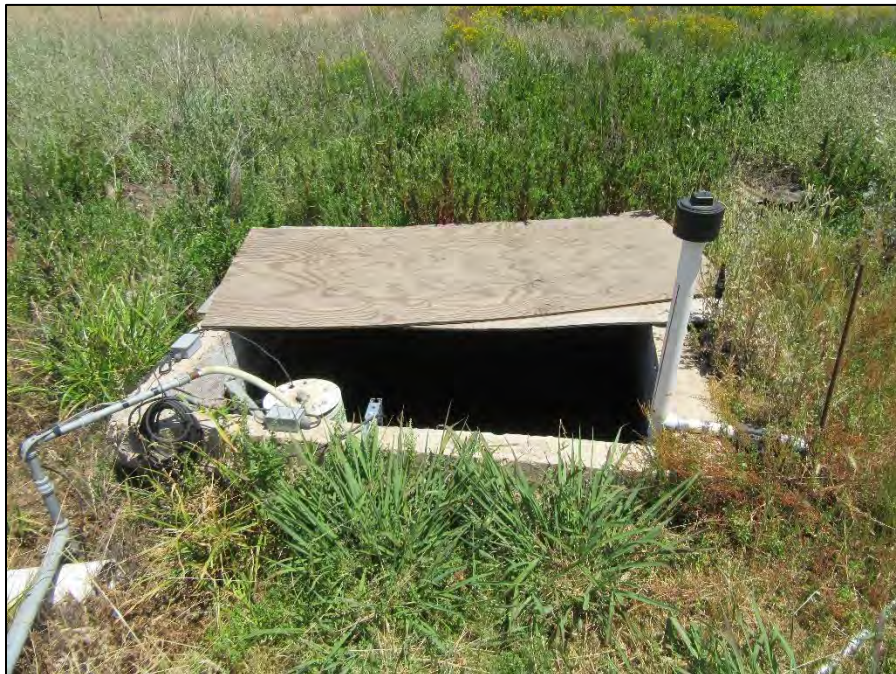
CC-02; well house overview (view north; May 27, 2022).
