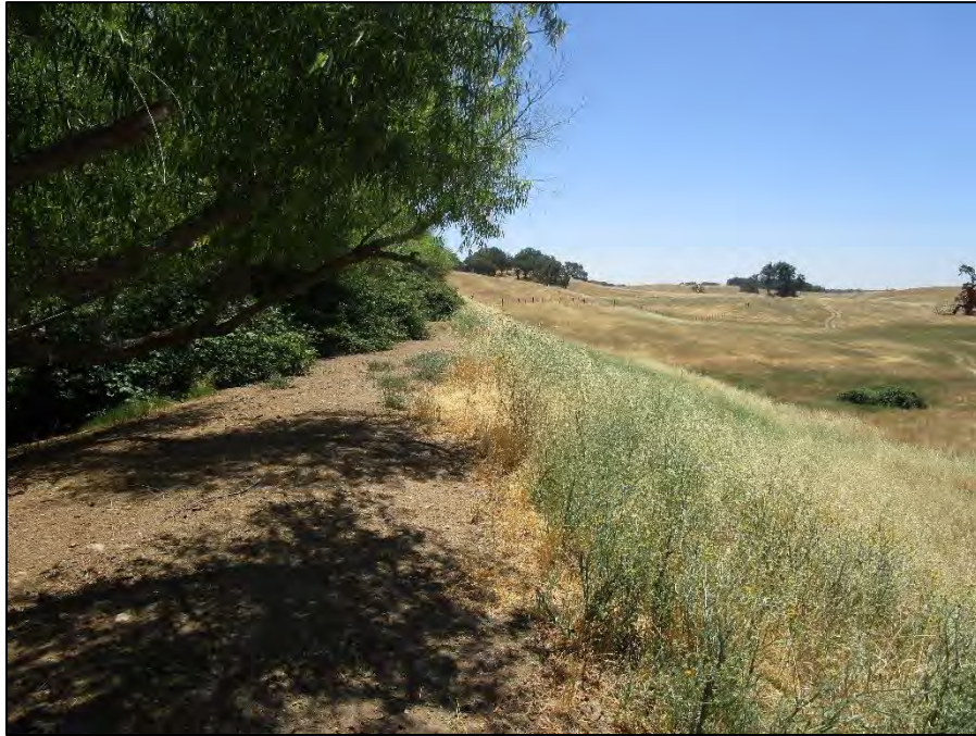
CC-07; earthen dam overview (view south; June 16, 2022).
