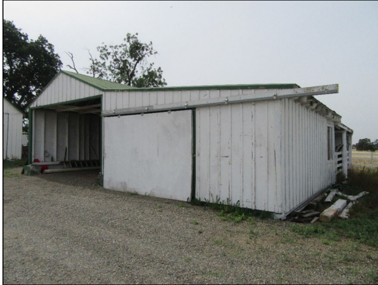
Figure 29. CC-01; Tractor Shed/Horse Stalls/Blacksmith Shop (view southeast; May 27, 2022).
