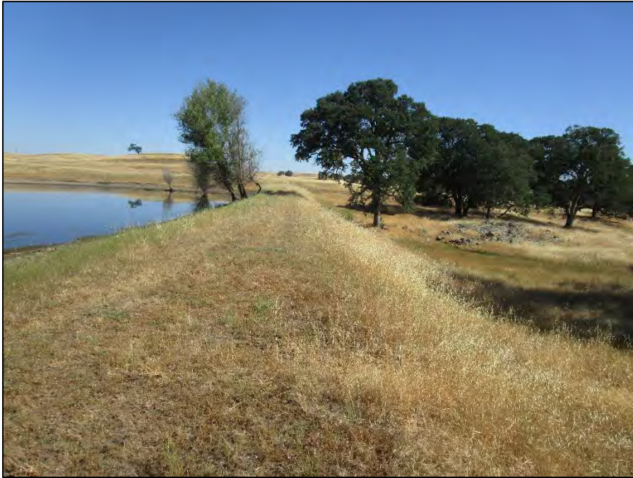
CC-08; earthen dam overview (view north; June 16, 2022).
