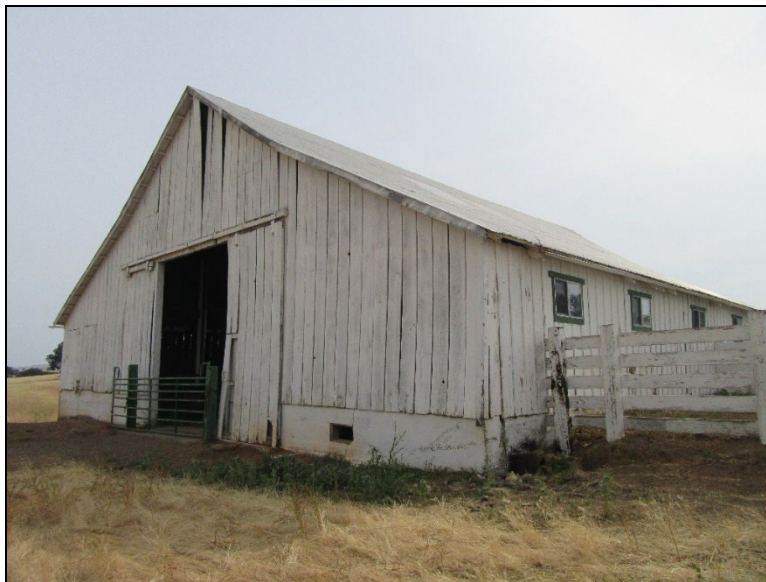
Figure 26. CC-01; Barn (view northeast; May 27, 2022).
