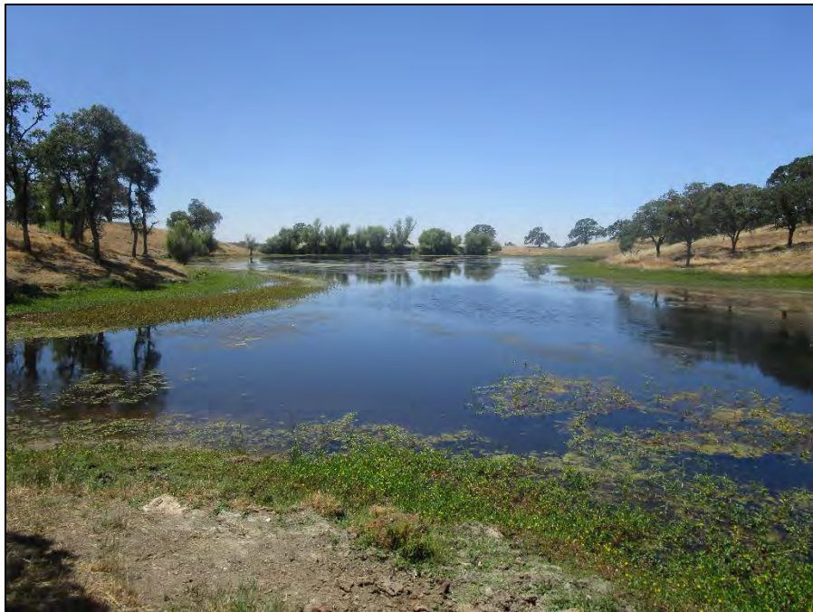
CC-07; earthen dam overview (view north; June 16, 2022).
