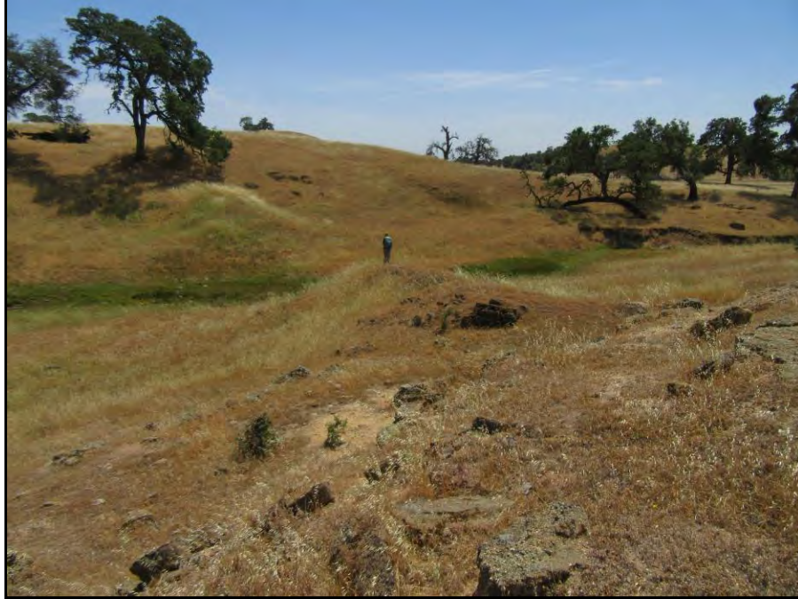
P-34-1577; earthen dam overview (view south; May 27, 2022).
