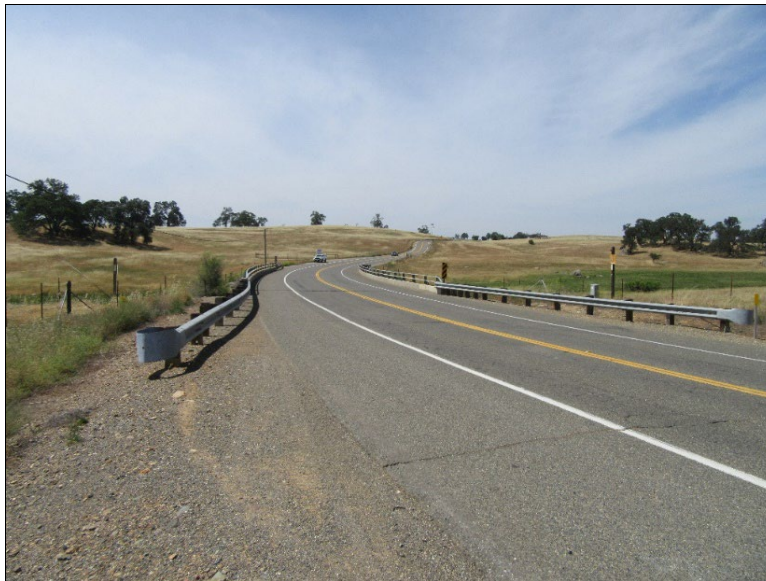
Figure 41. CC-03; Scott Road Overview (view north; May 27, 2022).
