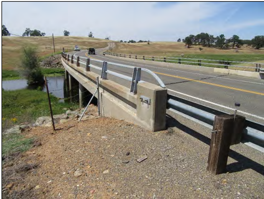
Bridge No. 24C0238 overview (view north; May 27, 2022).
