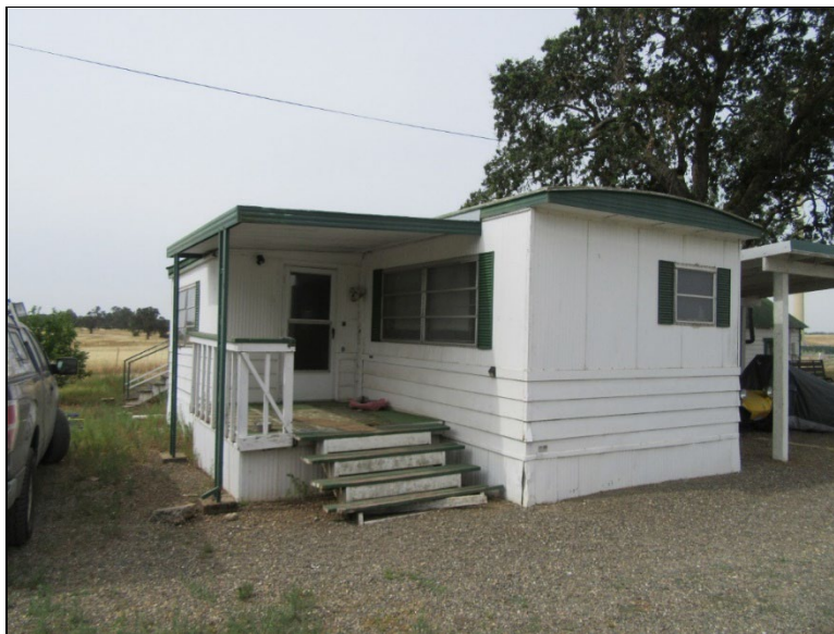
Figure 32. CC-01; Manufactured Home (view south; May 27, 2022).
