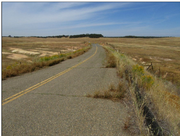
Figure 42. CC-04; Boys Ranch Road Overview (view east; May 27, 2022).
