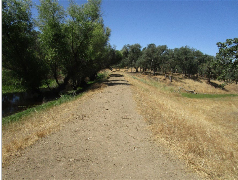
Figure 49. CC-10; Earthen Dam Overview (view south; June 16, 2022).
