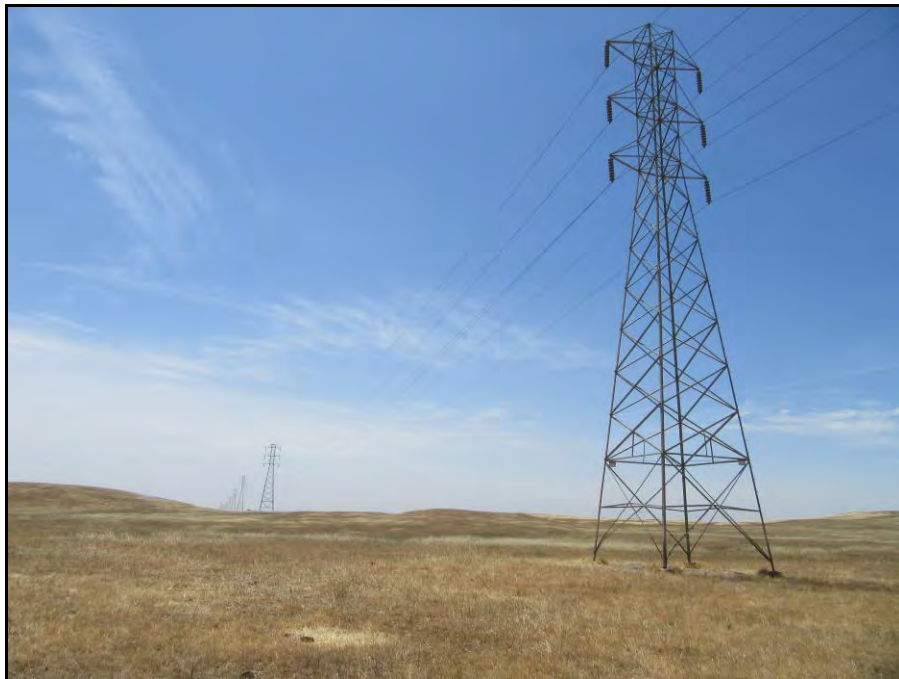
P-34-2195; Transmission line overview (view southwest; May 27, 2022).
