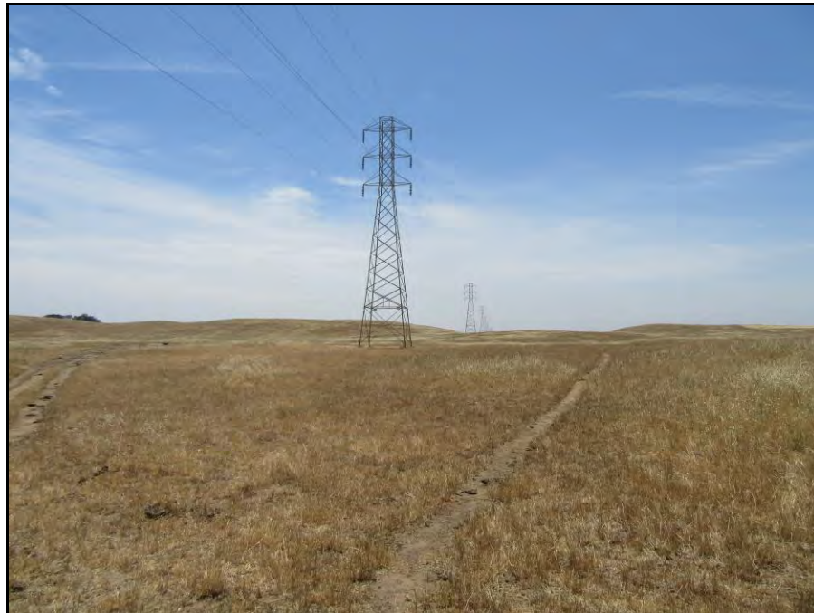
P-34-2195; Transmission line overview (view south; May 27, 2022).
