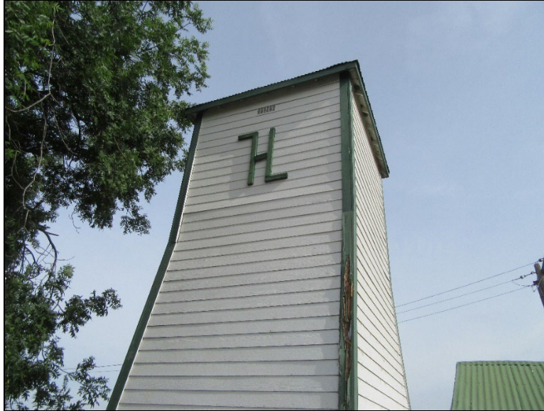
Figure 20. CC-01; Tankhouse (view northwest; May 27, 2022).
