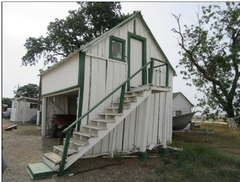
Figure 30. CC-01; Garage/Living Quarters (view southeast; May 27, 2022).
