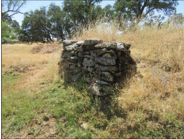
Figure 5. P-34-1575. Bridge Abutment on Coyote Creek Overview (view west; May 27, 2022).
