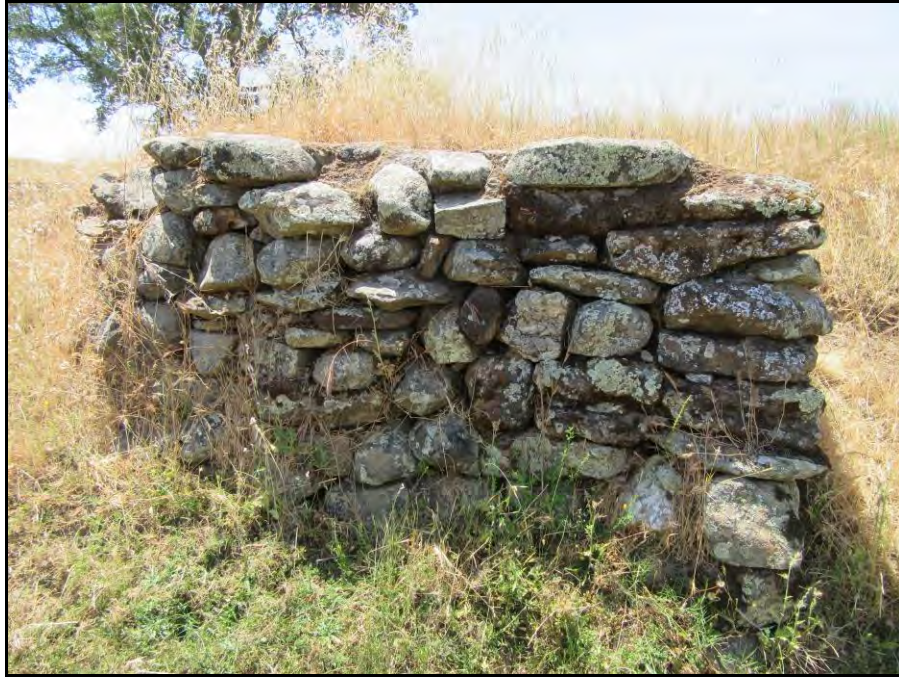
P-34-1575; bridge abutment overview (view east; May 27, 2022).
