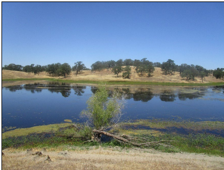
Figure 45. CC-07; Earthen Dam Overview (view north; June 16, 2022).
