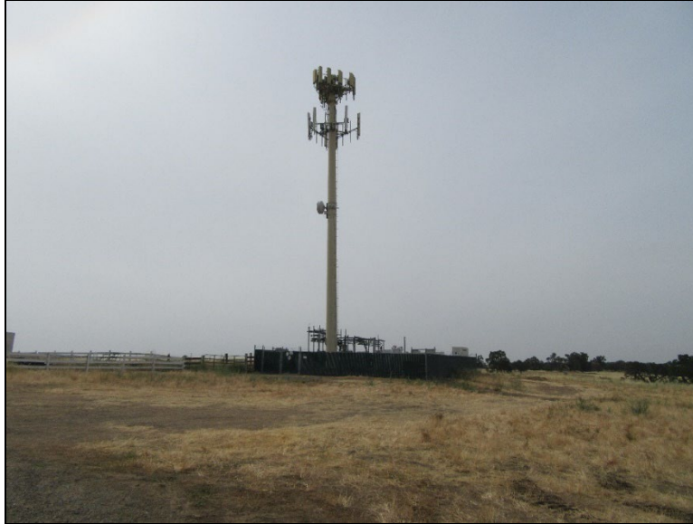
Figure 33. CC-01; Cell Tower (view southwest; May 27, 2022).
