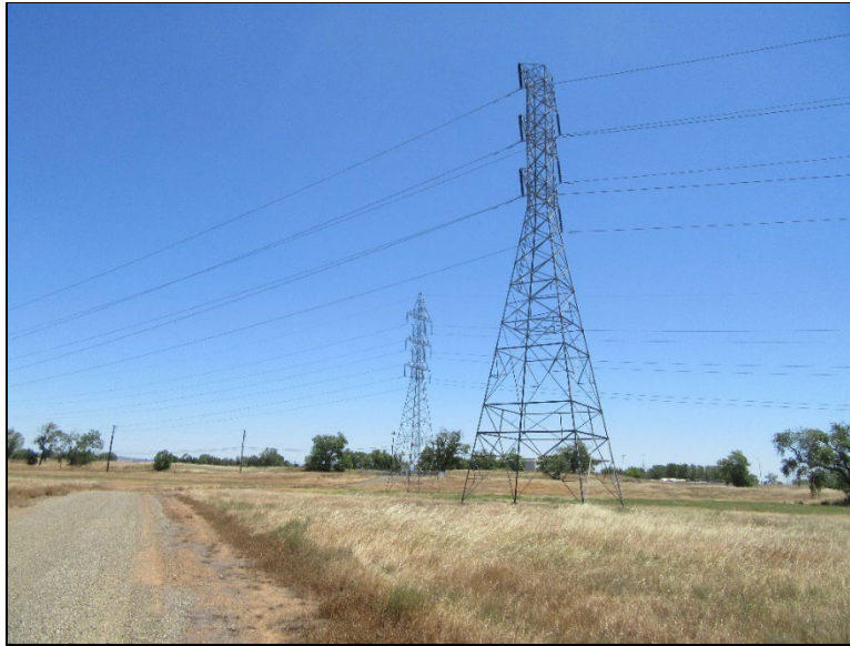
Figure 13. P-34-5267 and -5268; Transmission Line Overview (view east; May 27, 2022).
