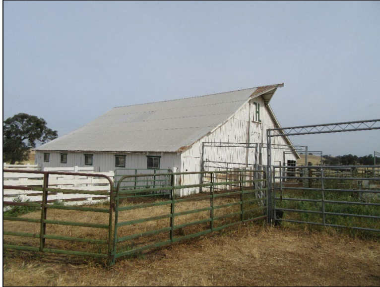
Figure 25. CC-01; Barn (view northwest; May 27, 2022).
