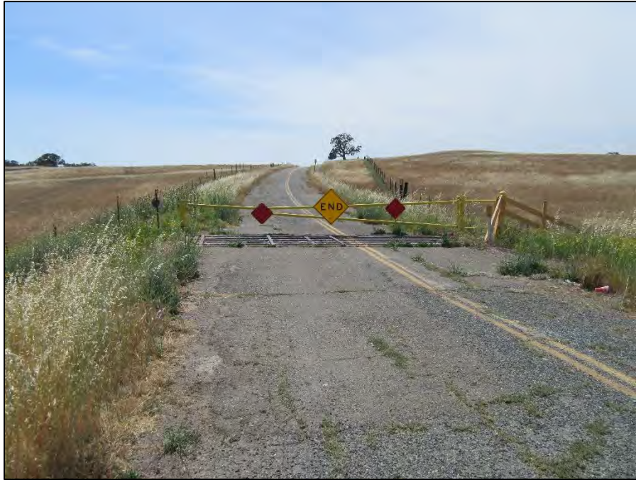
Boys Ranch Road overview, view to school (view west; May 27, 2022).
