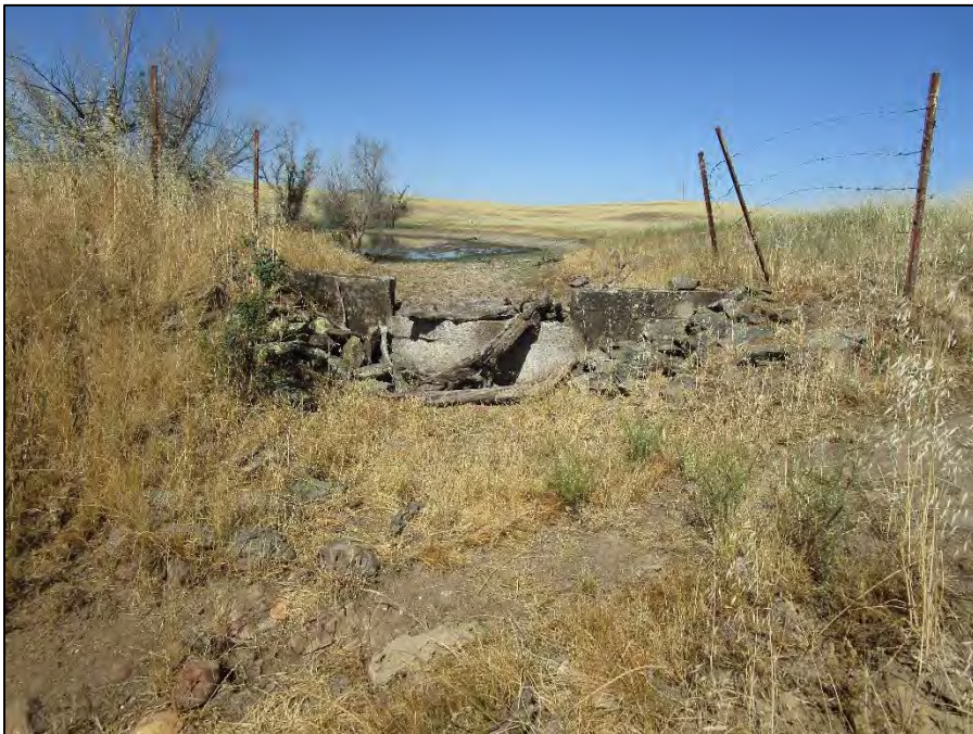
CC-08; reservoir overview (view west; June 16, 2022).
