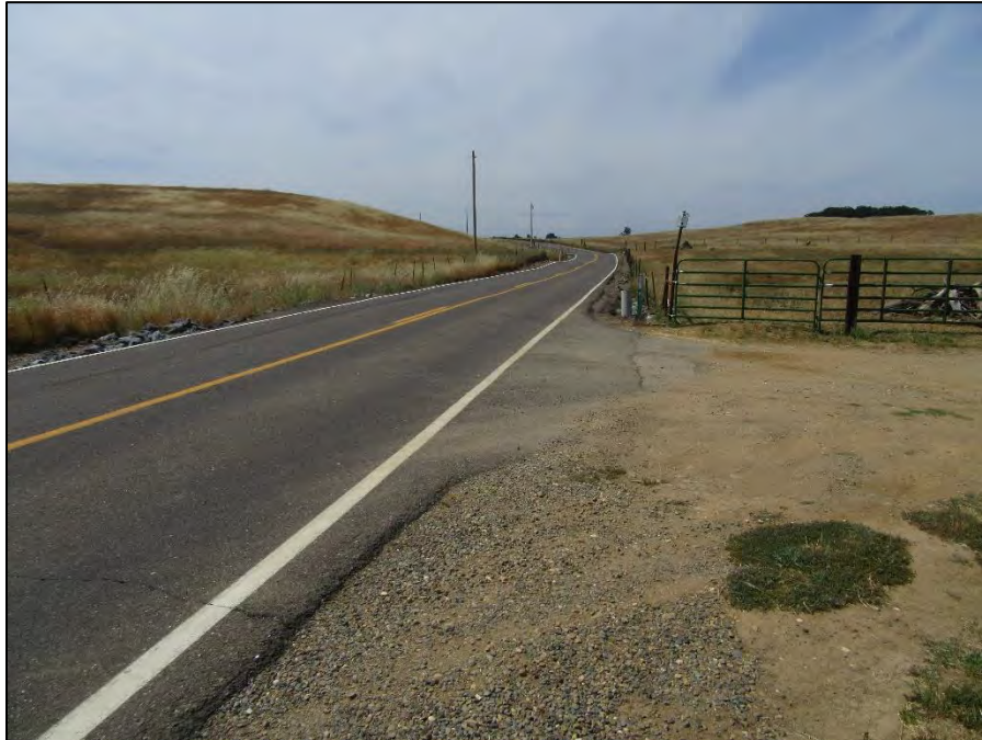
Scott Road overview (view north; May 27, 2022).
