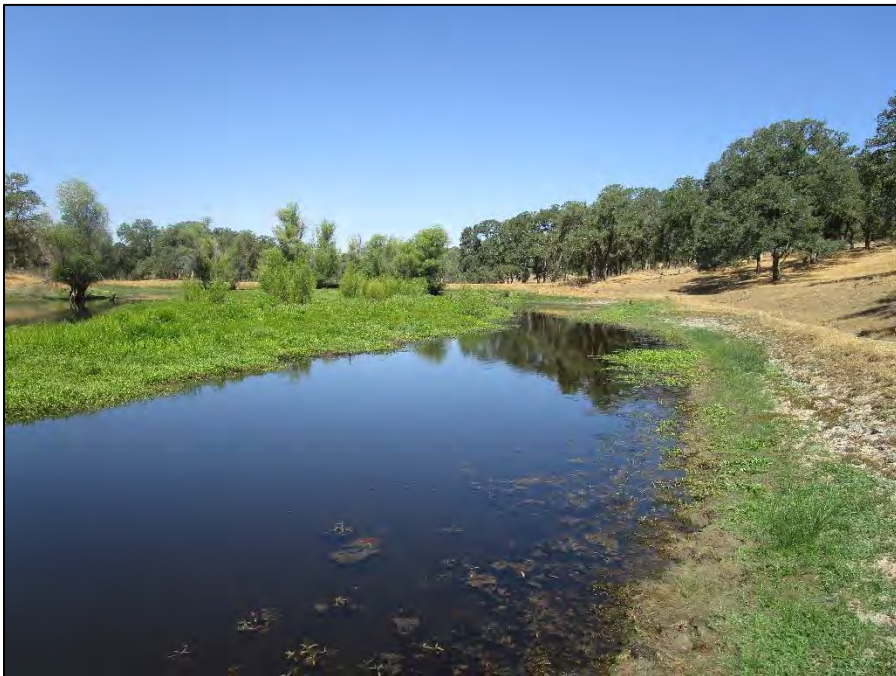
CC-10; reservoir overview (view west; June 16, 2022).
