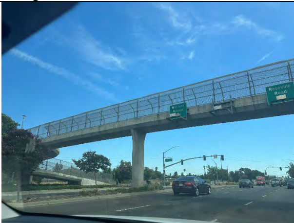
Developed land cover with deep holes under bridge, suitable for nesting birds and bats, north of intersection of Peacekeeper Way and Watt Avenue, facing south.
